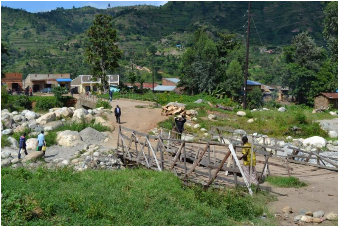
Kyarumba town, Kasese district, Uganda: In the foreground, a newly constructed temporary bridge following floods, with a permanent bridge in the background ( source: Nikhil Advani )
